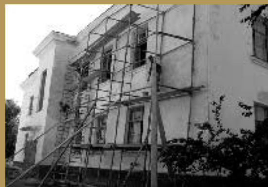
Chat Bazarr Hospital Refurbishment – Talas region
