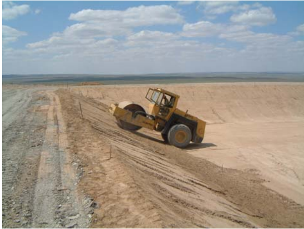
Raw Water Dam
