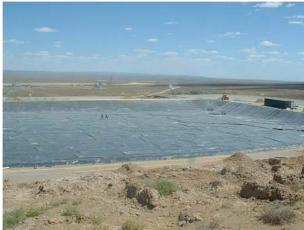
Raw Water Dam
