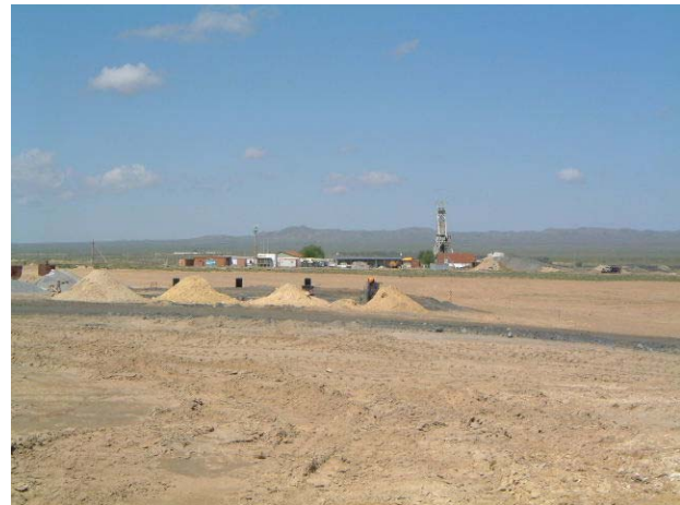
Plant Site Preparation
