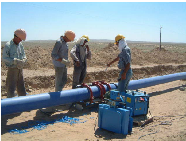
Raw Water Pipeline
