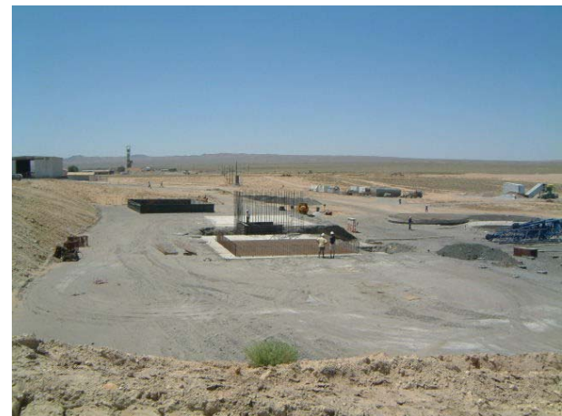
Plant Site Preparation
