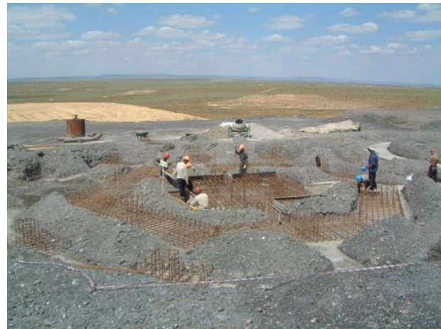
Plant Site Preparation
