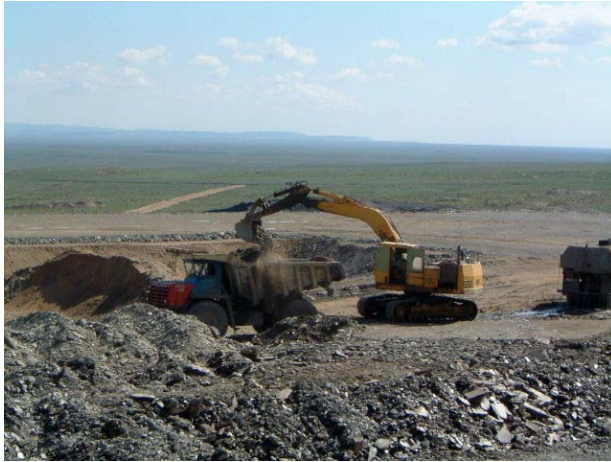
Raw Water Dam
