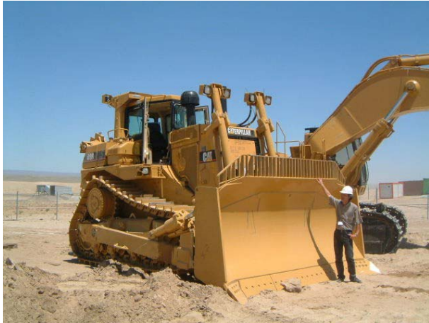
Machinery arriving on site
